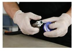
5) Dry the solvent from the ends of the mixing tube and whip hose and apply Teflon tape to the threads.
