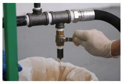
8) Purge the pressure release ball-valve during the flush process.
