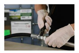
10) Attach, the whip hose and tighten all connections.
